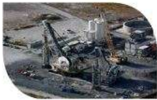
Ultra Deep Diaphragm walls
