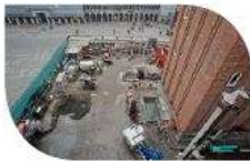
Ground Consolidation San Marco Square - Venice Italy
